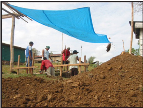
Parents and Caracoles excavating for the septic tank
